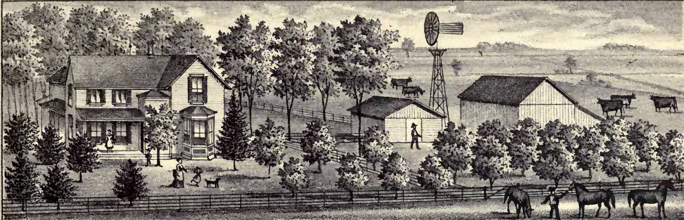
RESIDENCE OF L. MASON , SEC. 12. PONTIAC TOWNSHIP.
